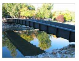
Acciona Infaestructuras S.A and its partners have designed and manufactured a composite bridge beam made from a single piece (40 m long) and weighing only 25 t, which is half the weight of a concrete or steel bridge (minimum 50 metric tons). The beam required a "slenderness ratio" (ratio of depth to the length of the beam) of less than 1.2/40, combined with a maximum cross sectional thickness of 50 mm and a depth of 1,200 mm.
