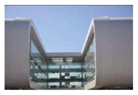
The concept is based on a large folding skin wrapped around the modules containing the rooms. This outer skin is made of glass-fibre-reinforced composite material. The final solution uses a damp-proof reinforced membrane finished in white for the flat roof, combined with a pultruded glass-reinforced plastic sheeting on a metal sub-structure for the curves and the down-stands of the skin.
